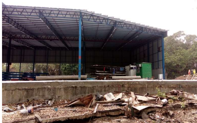
Photo 2.12 Inactive Brownfield Sites
