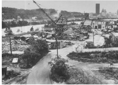
Photo 7.1 Brownfields of Pittsburgh in 1960s Source: © Urban Redevelopment Authority of Pittsburgh
